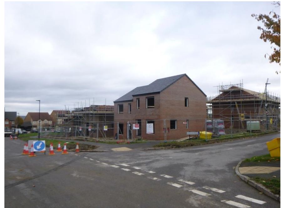
New Council houses in development on the Weakland estate
