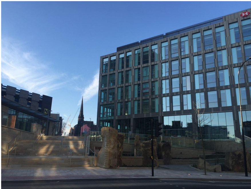
A new, vibrant city centre in development as part of our ‘Heart of the City II’ project – the HSBC building
